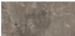
WEATHERED AGGREGATE (G)
